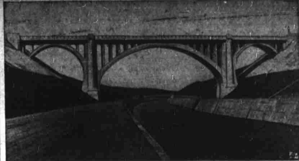
FOR WAR AND PEACE, Belgium is building the Albert canal, connecting Liege and the Meuse river valley, in the east, with Antwerp on the west near the North sea. This is the canal bridge at Vroenhoven. The canal will accommodate boats of 2,000 tons and will have six giant locks to raise or lower them. The elevation between Liege and Antwerp changes 195 feet.
