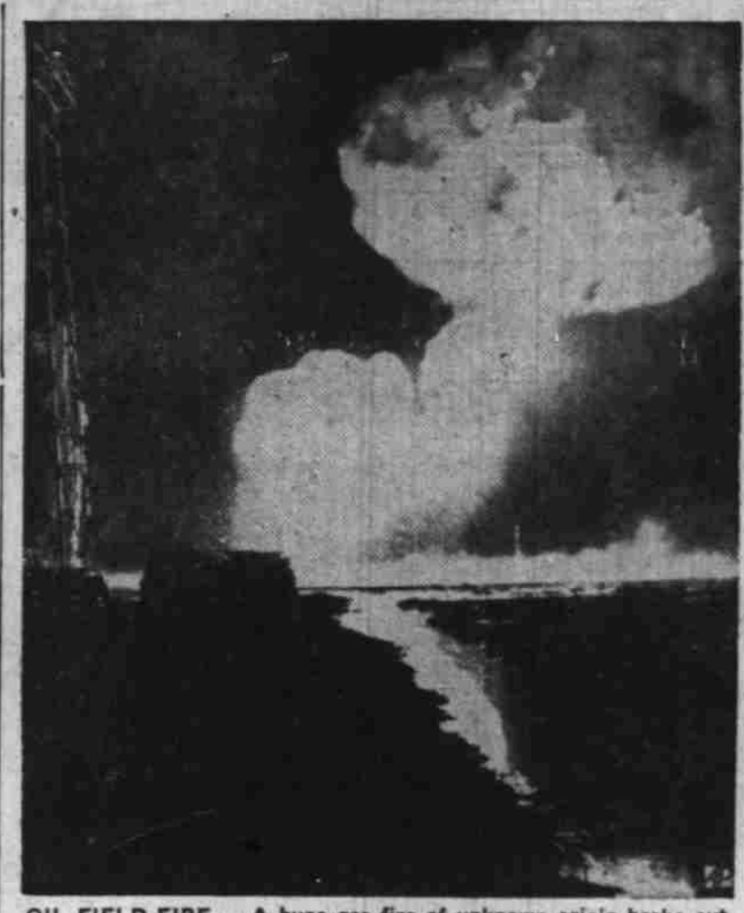
OIL FIELD FIRE — A huge gas fire of unknown origin broke out between two oil wells in the South Houston, Texas, oil field, during the night of March 23.
