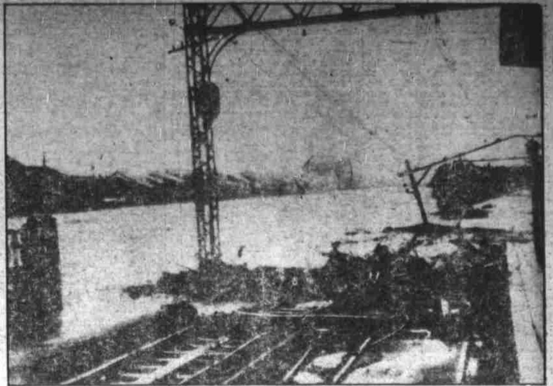
At least 91 persons were killed in western and central Japan in sweeping floods that swept over the district. Damage was estimated at more than 10,000,000 yen. The photo shows Hankyu station, main outlet for Kyoto's heavy interurban traffic, which was wrecked by the high waters. (Associated Press Photo)
