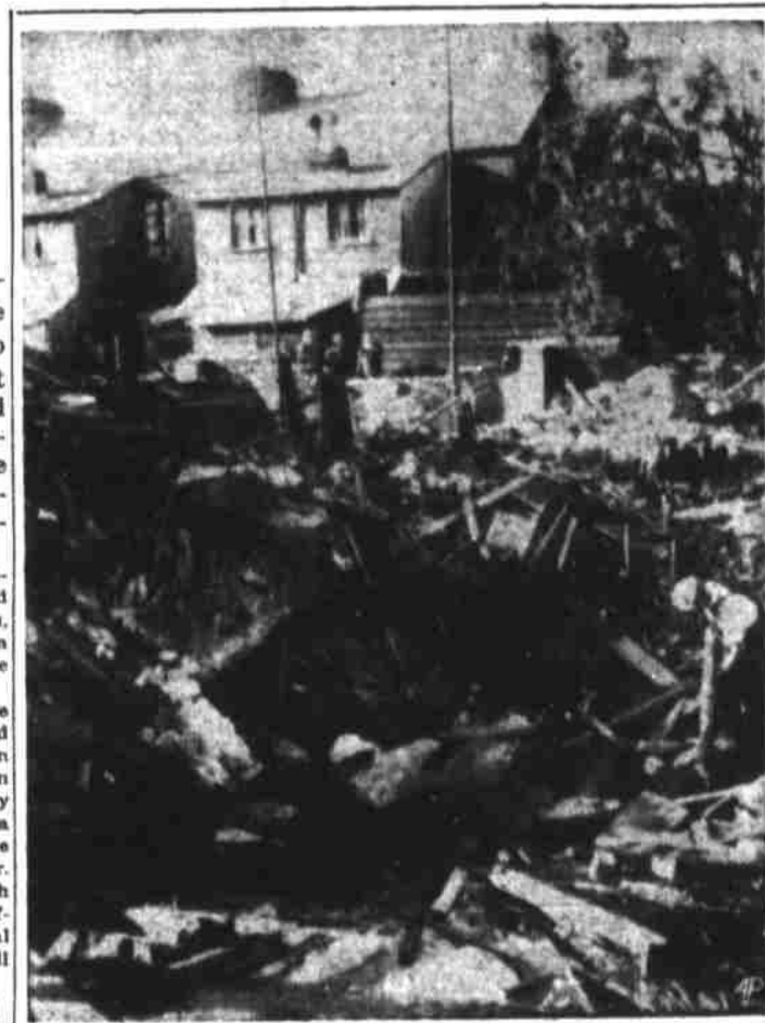
WAR STRIKES THE TIGHT LITTLE ISLE—This pile of ruins once was a house in Cambridge, England, according to British sources. This damage was a result of German bombs dropped June 19. Since then, naval planes have raided towns in the north-eastern coastal section, causing casualties in the hundreds.
