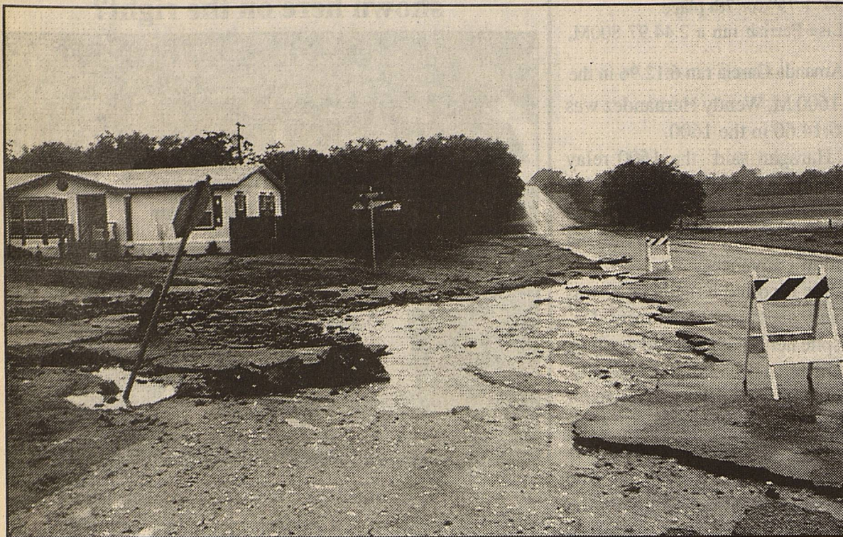
Several streets around town were damaged by runoff water following the rain, including this one in front of the Jack Lowe residence.
