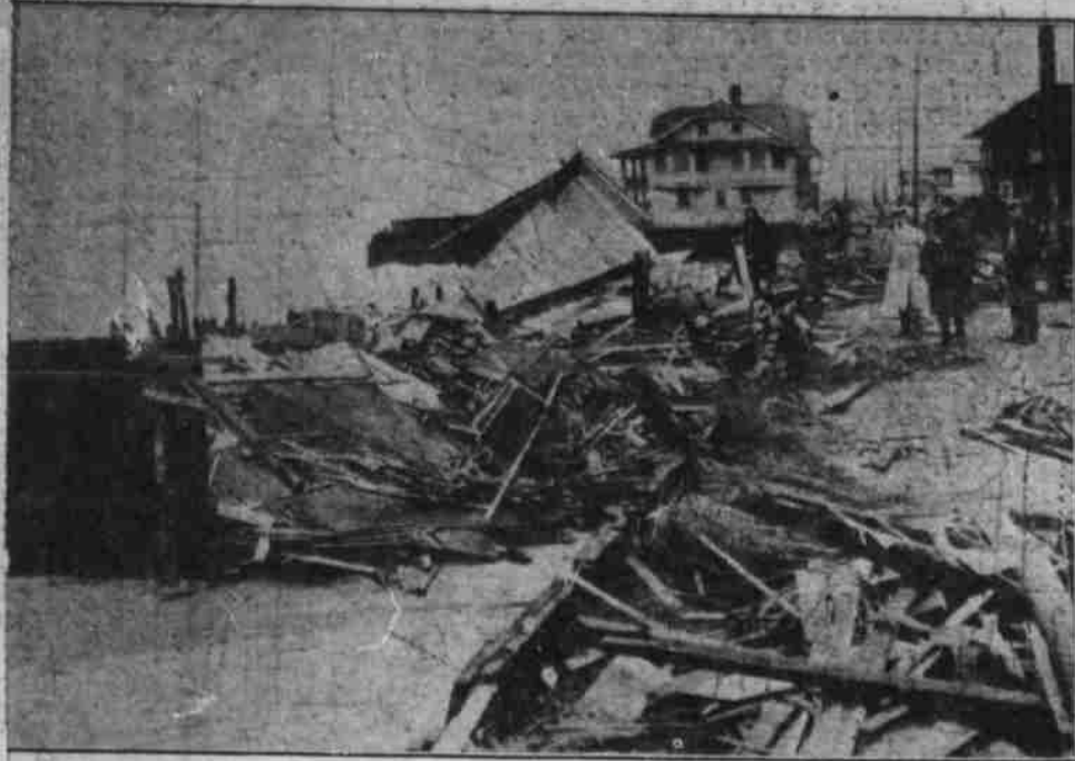
A 60-mile-an-hour gale that roared in from the ocean hammered the coast from New York to North Carolina causing thousands of dollars worth of property damage. The Jersey coast was most severely hit. Huge seas piled up by the wind raked the shore resorts washing tons of sand from the beaches, undermining cottages, and flooding streets. Above is the ruins of a summer home at Ocean City, N. J. (Associated Press Photo)
