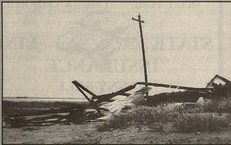
This barn belonging to Larry Rawls on the Allred Road was hit by extremely high winds in last Tuesday's bout with heavy rain and reported tornados in the area.
