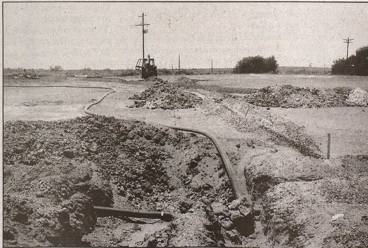
Top photo shows employees digging ditches for natural gas and electric lines to dryer site, photo below shows lines to be routed and buried at Attebury-Williams Peanut plant
