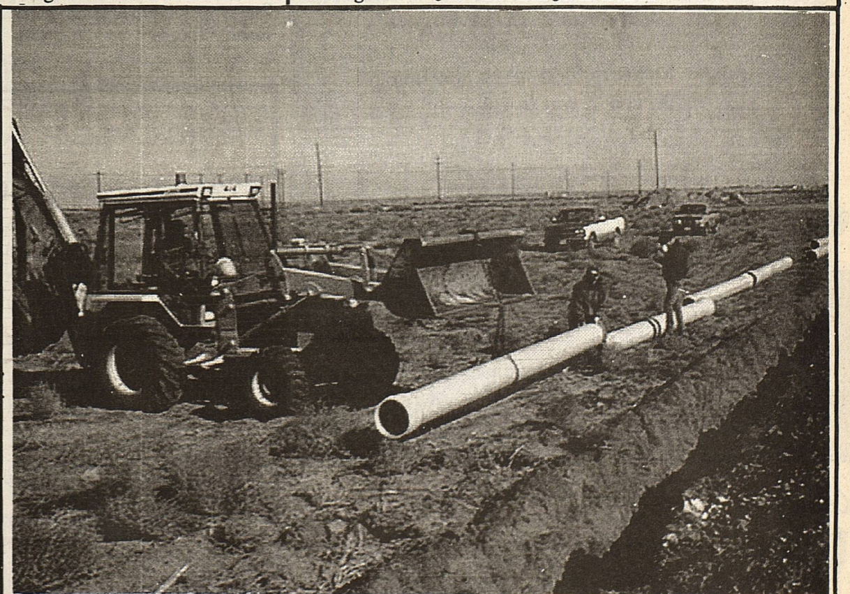
Alex Barrientes, on backhoe, unloads PVC pipe for waterline project
