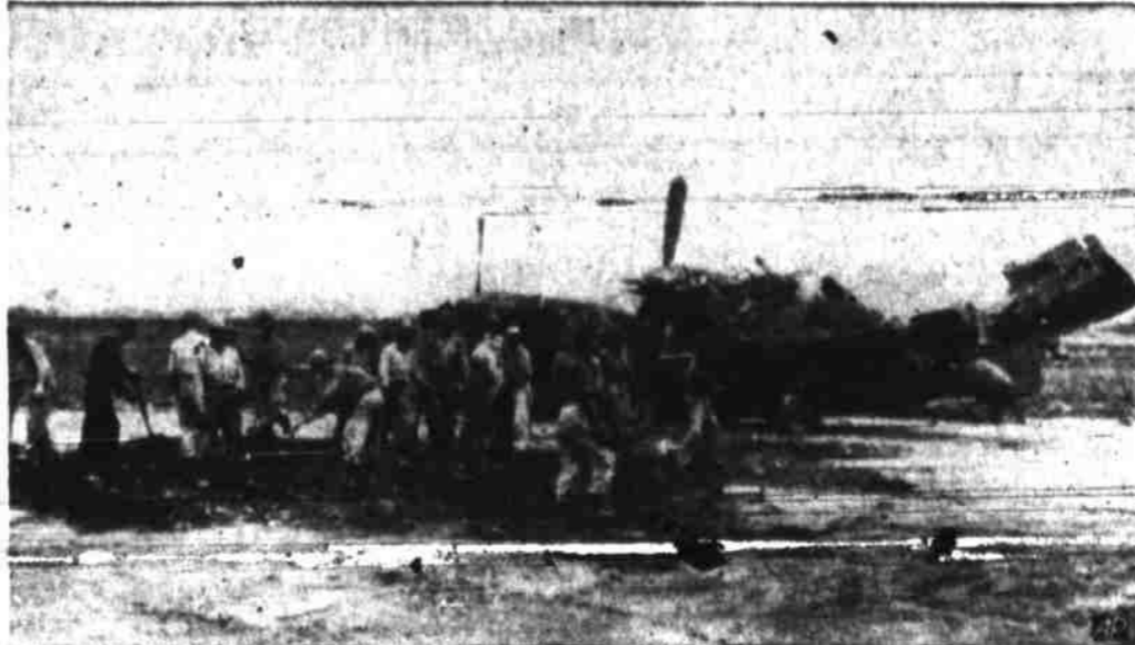
BOMB DAMAGE REPAIRED AT SUWON AIRFIELD—These Korean soldiers repair damage inflicted by Russian-built Yak fighters in strafing and bombing attacks on Suwon Airfield in Korea. A damaged F-82 plane is shown in the background. This picture was made by C. P. Gorry, Associated Press staff photographer. (AP Wirephoto).
