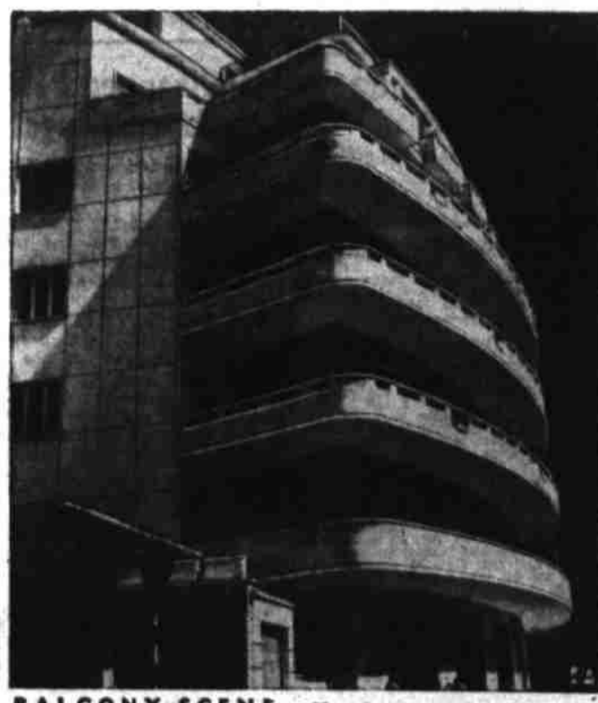
BALCONY SCENE — New houses mushrooming all over Rome, Italy, provide visitors a three-room apartment with flowered modern-type Juliet balconies like these for $65 a month.
