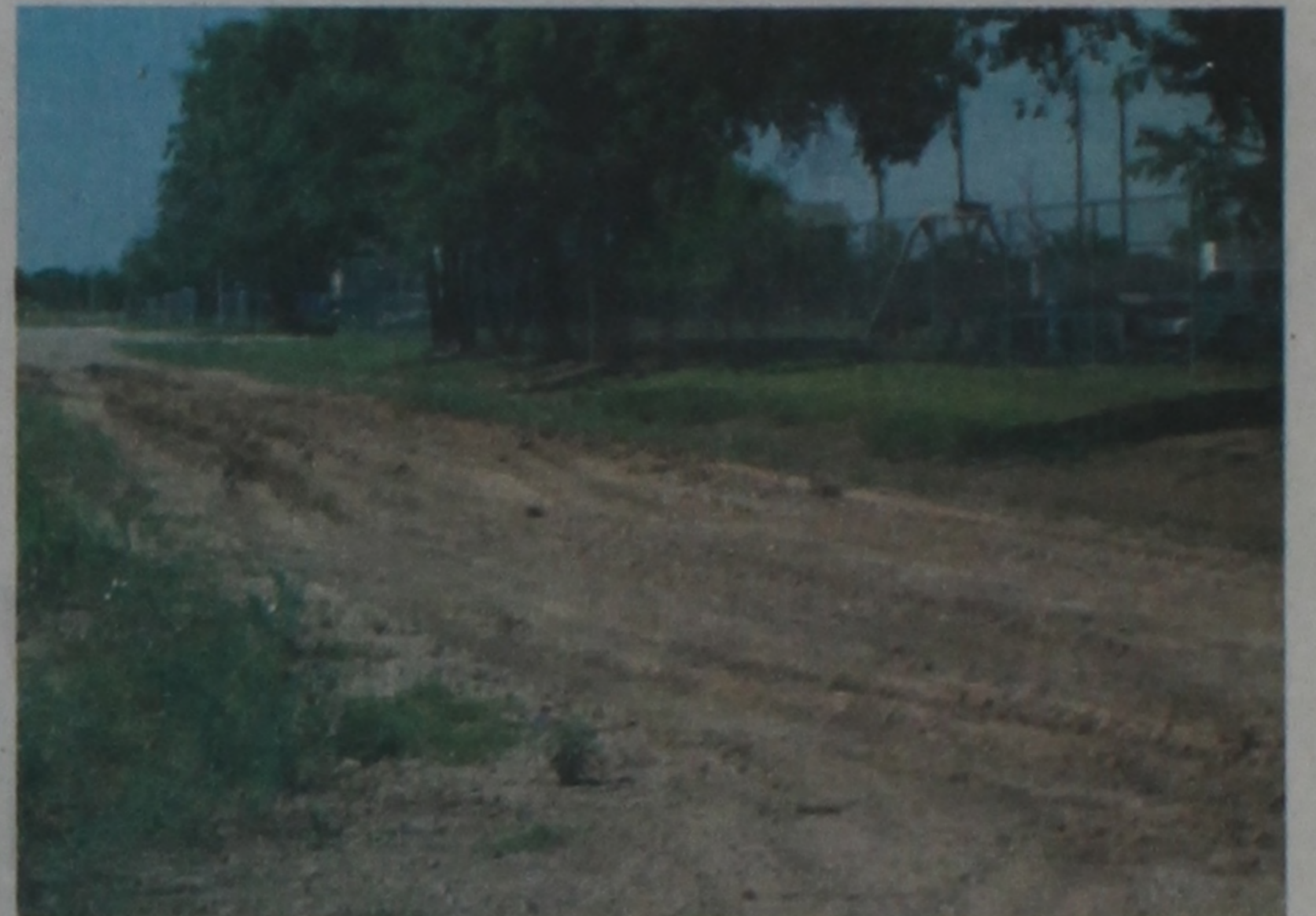
Dirt road at East East 16th and Idalou Road
