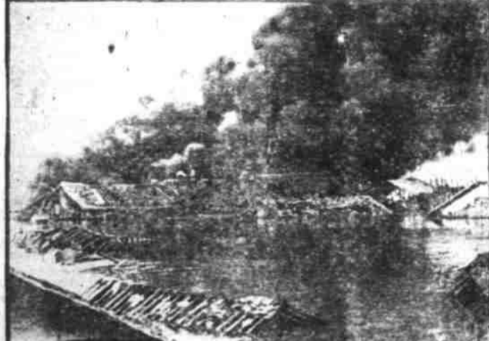
The Looe River, showing a Chinese village almost inundated by recent floods, was typical of the view obtained by Col. and Mrs. Charles A. Lindbergh as they flew over the Chinese flood area. At Hankow, where floods caused widespread tragedy, a fire (below) destroyed an American oil company's huge storage plant.
