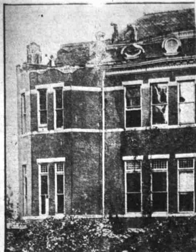
A local tornado caused about $10,000 damage when it hit Columbia, Mo., and swept a turret off Swallow hall, University of Missouri Geology building. Workmen are shown repairing the roof.
