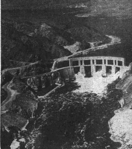
CALLED THE BEAUTY QUEEN AMONG DAMS, the 280-foot-high Parker dam on the Colorado river, 155 miles below Boulder dam, is shown above in a recent view. Two-thirds of its height is submerged. Parker is the diversion dam for the 242-mile aqueduct built to carry one billion gallons of water a day for the domestic needs of Los Apreles and 13 nearby cities.
