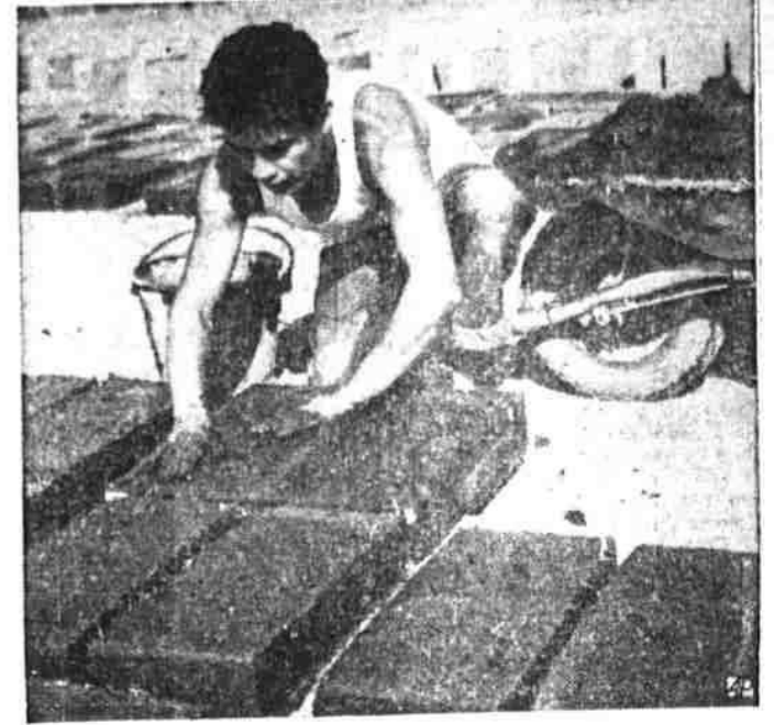
BRICK BUILDER Carlos Martinez, CCC youth who is helping restore mission near Lompoc, Cal., to its 19th century glory, carefully molds adobe bricks for use in the restoration. Wooden mold gives the bricks their shape. One minor tragedy among the CCC brick-makers was the loss of some 5,000 adobe bricks left in the sun to dry; a rainstorm melted them all.
