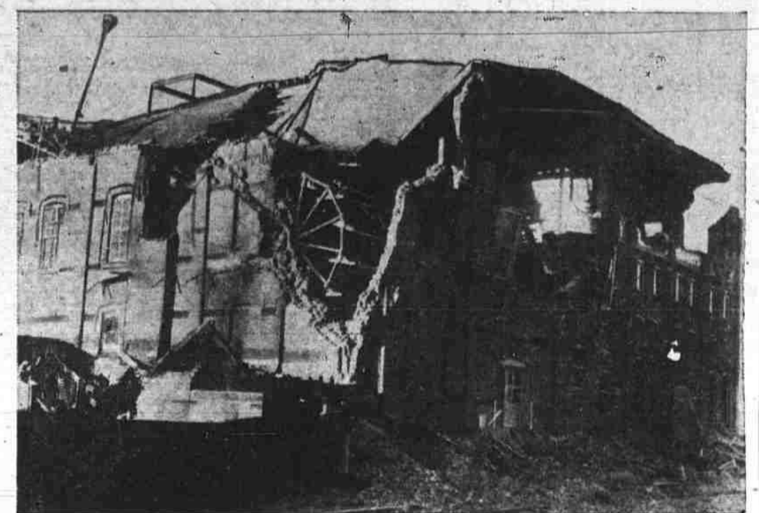
Two persons were killed and damage estimated at a million dollars was caused by the terrific force of an earthquake which struck Helena, Mont. Above may be seen the ruins of the National Biscuit company warehouse, one of the buildings in the town which was badly damaged. The walls of the structure were shattered by the tremors. (Associated Press Photo.)
