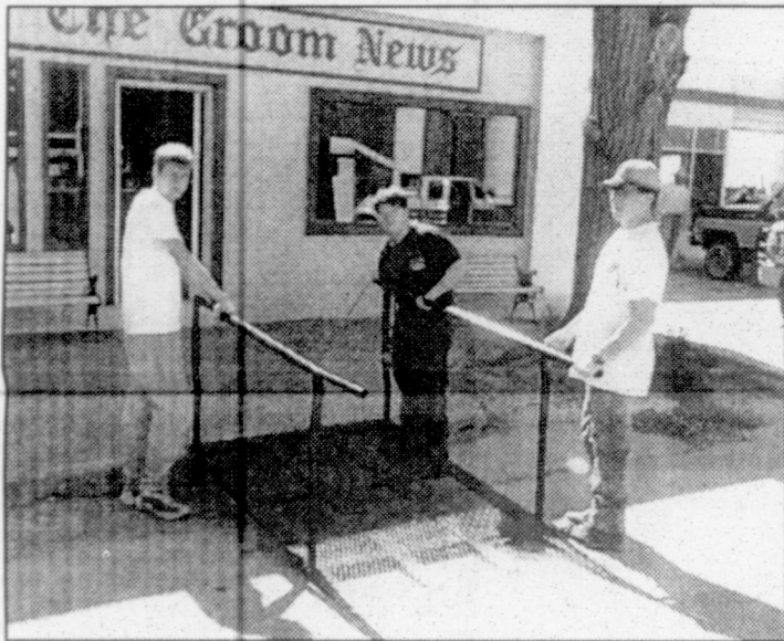
James Ratteree, Cody Britten, Dennis Cockrell and teacher Charles Burk unload a very welcome ramp in front of the News office. The Ag/Welding students have done several public service projects for the school and city.
