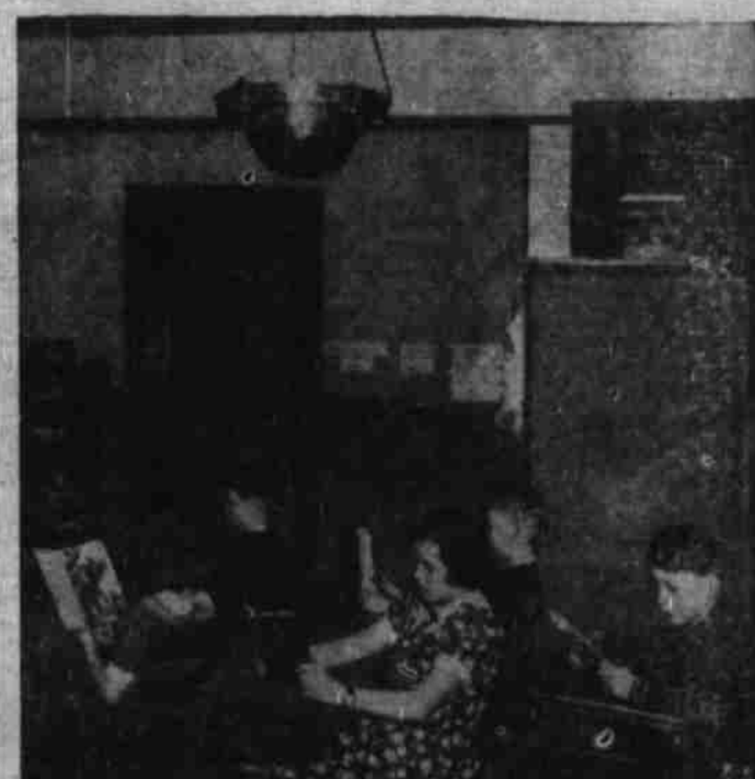
GERM-FREE AIR for school pupils is goal of University of Pennsylvania scientists directing installation of a new lamp in this junior grade room at Germantown Friends school. From the lamp, invisible ultra-violet light radiates, cleansing the atmosphere—it is believed—of harmful bacteria.
