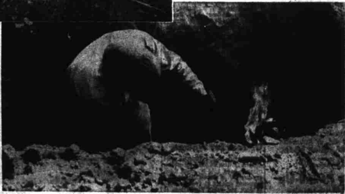
Welder is Tying In New Line As Part Of Empire Southern Expansion Work
