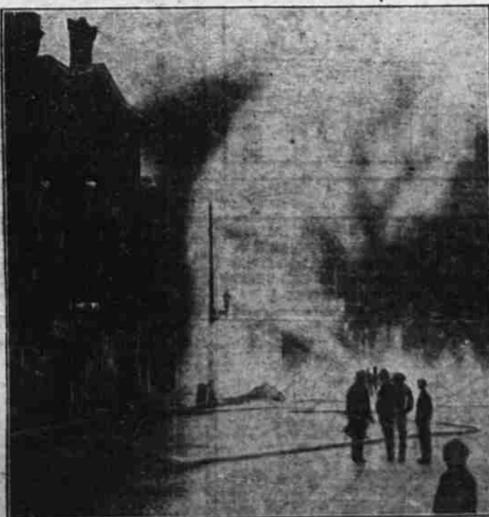
Associated Press Photo Five buildings were destroyed and six others damaged by a fire that threatened the entire business district of LaGrange, Ga. Damage was estimated at $400,000 to $750,000. Firemen from five cities fought the blaze.
