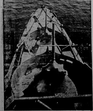
Navy destroyer-escort, attached to the inactive "sipped-up" for peace, at Green Cove Springs, Fia. against rust, the two forward gun mounts are special coverings made of special plastic.
