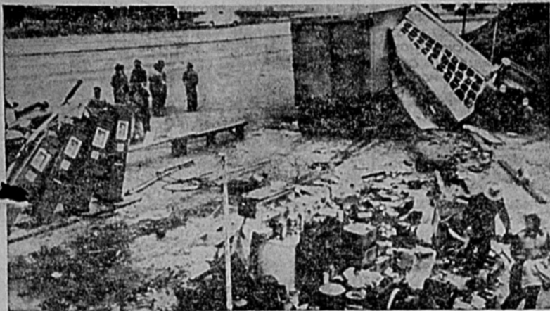
BRISBANE, CALIF.—(Soundphoto)—Tilted gas pumps and mass of debris are all that is left of steel-frame gas station here after it was hurled off its foundation and carried 20 feet when a huge 18-wheel truck-trailer veered off Bayshore highway and smashed through it. John Vincequerra, 24, San Jose Calif., the truck driver, said two automobiles in front of him suddenly stopped directly in his path. He applied airbrakes, but they failed, and he swerved to avoid hitting the cars. The truck plunged across curbing and into gas station, carrying it with it before coming to rest (rear) against hill.
