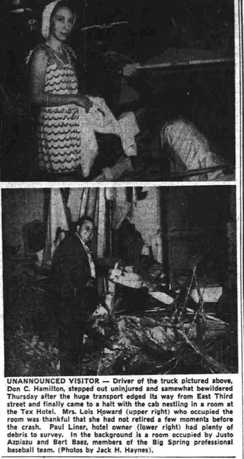
UNANNOUNCED VISITOR — Driver of the truck pictured above, Don C. Hamilton, stepped out uninjured and somewhat bewildered Thursday after the huge transport edged its way from East Third street and finally came to a halt with the cab nestling in a room at the Tex Hotel. Mrs. Lois Howard (upper right) who occupied the room was thankful that she had not retired a few moments before the crash. Paul Liner, hotel owner (lower right) had plenty of debris to survey. In the background is a room occupied by Justo Azpiazu and Bert Baez, members of the Big Spring professional baseball team. (Photos by Jack H. Haynes).
