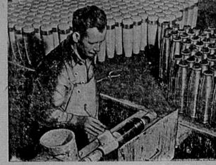
Shaving a 7.2 inch howitzer shell on a giant lathe. The Dom--25-pounder: 3.7-inch anti-aircraft: 4.5-inch; 6-inch how- inion's ammunition factories make 18 types of shells in 14 different calibres. They employ 50,000.
