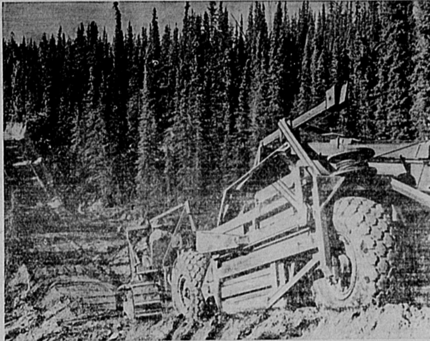
On this carry-all tons of earth were moved from a high section to fill a low section of the Canada-Alaska Highway. Hidden two or three feet under the muskeg in some sections are glacial ice formations thousand of years old. When the muskeg is removed the ice melts, creating heavy morass, but the U. S. Army engineers have found a solution to the problem.
