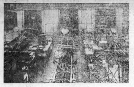
THE Buick Motor Company has announced the completion of its new, efficient assembly system, the Unified Line.
