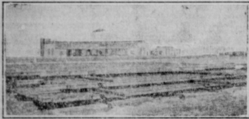
This picture was published in The Slatonite Sept. 20, 1912. It shows the Santa Fe round house and machine shops which had then been completed. The construction was of re-inforced concrete and so arranged as to double the size when needed.
