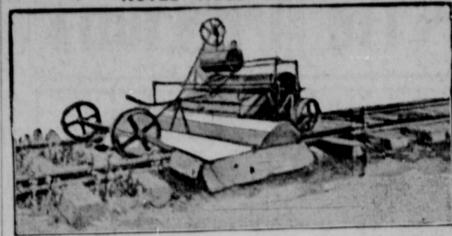
Stretches of Track Can Be Cleared of Weeds in a Day's Time With This Burner, Which is Pushed Slowly by a Locomotive.
