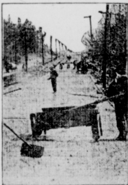
Vitrified Brick Pavements for Country Roads—Filling the Joints.
