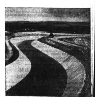
FOR THIRSTY LAND\_Part of the 37-mile-long Madera Canal, which will carry water from California's Friant dam to the Madera irrigation district winds in a S-curve through foothills. Dam is 35 feet wide at the top and 10 feet deep.
