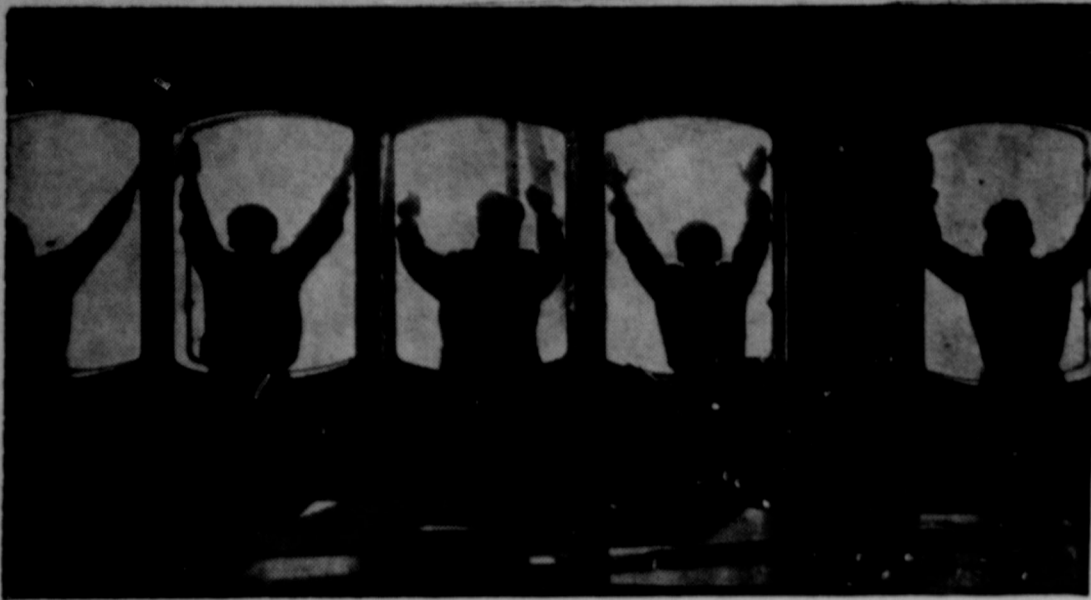
REACHING FOR THE SUN —These shadowy figures, silhouetted against the bright windows, aren't prisoners looking to escape, but glaziers fitting glass panes. They're working on the uppermost deck of the Swedish-American luxury liner Gripsholm. The 23,000-ton ship is being readied in Genoa, Italy, for its maiden voyage to the United States next summer.
