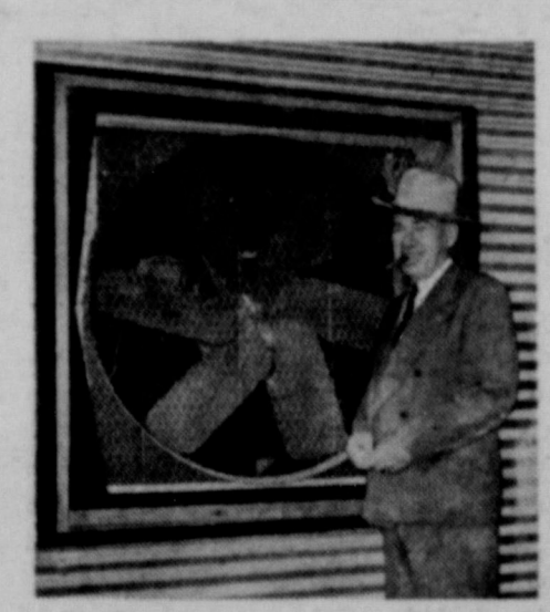
Mr. Art Chesher of Littlefield expects the pad and fan cooling system to increase production as much as 20% and reduce layer culling 12%.
