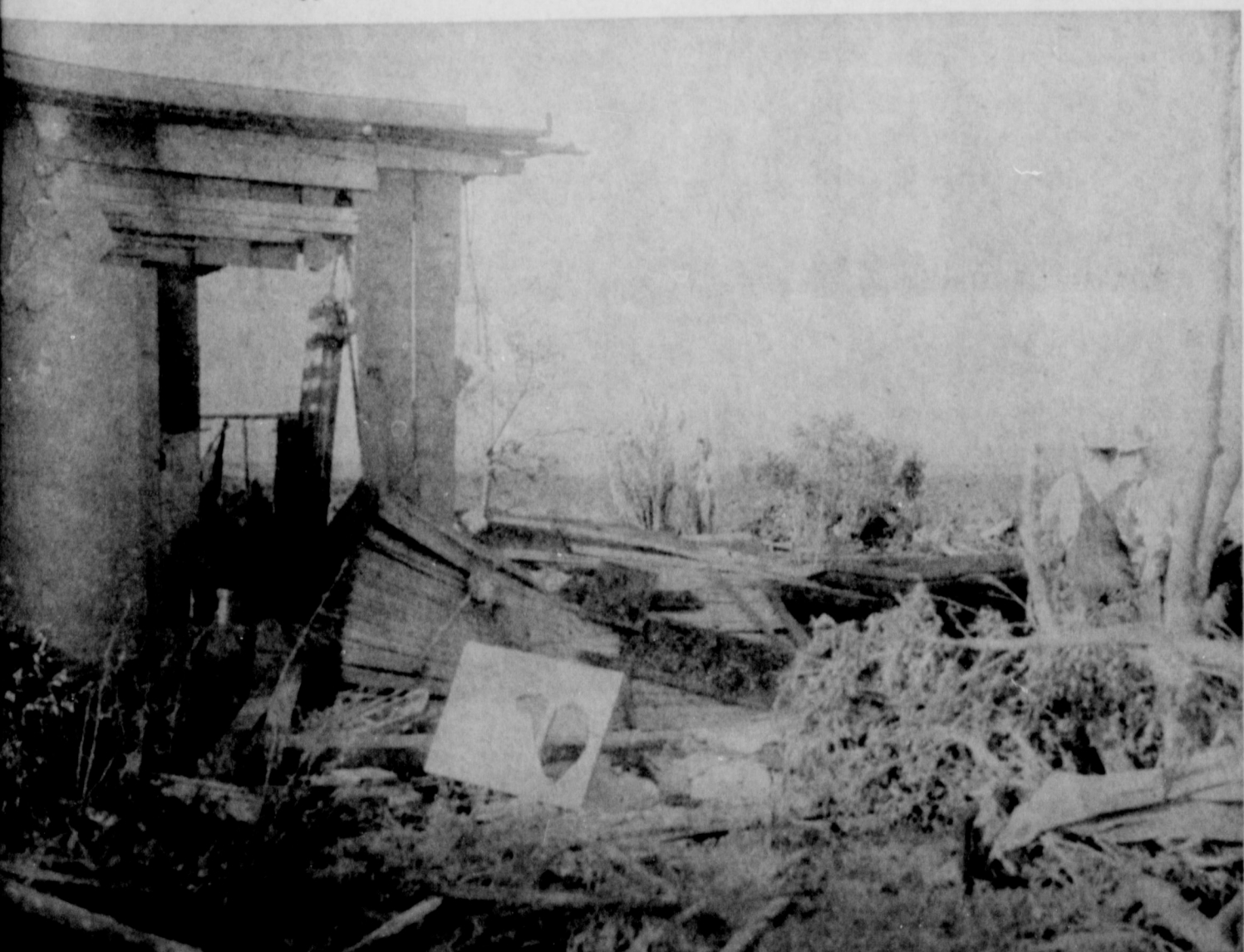
SOUTHWEST CORNER PROTECTION —Freakish as it might sound, the southwest corner of houses that weren't completely destroyed were about the only parts that remained. Civil Defense authorities advise it is safest to take shelter in the southwest corner of a house, under a bed, if you are unable to take shelter in a storm cellar. (SLATONITE STAFF PHOTO)
