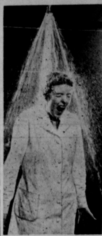
SAFE, ANYWAY —Chemistry technician Glenda Bates is doused for safety's sake. She's demonstrating the emergency shower for workers whose clothes become splattered with chemicals or catch fire. Similar showers are spotted around this chemical laboratory of the Parker Pen Company in Janesville, Wis.
