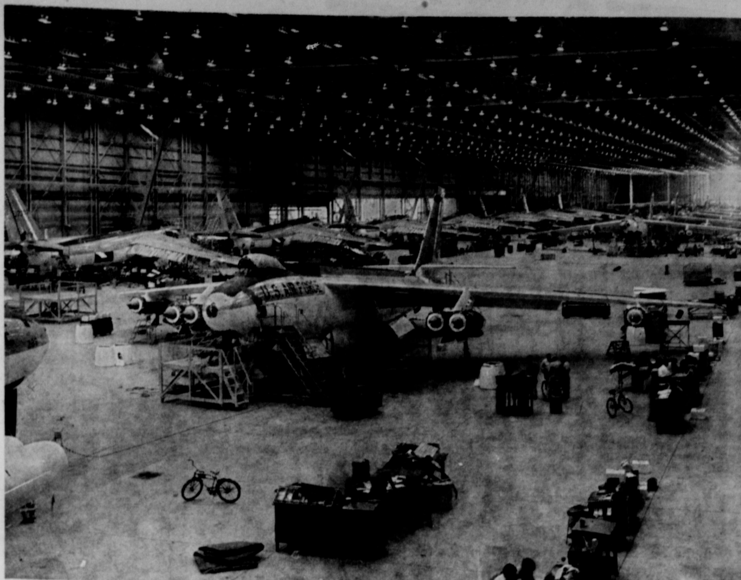
THIRTY-SIX B-47 BOMBERS can be repaired simultaneously inside the new $14,000,000 aircraft maintenance hangar at Kelly Air Force Base, San Antonio. The building is 2,000 feet long, 300 feet wide, and 92 feet high. It will accommodate
