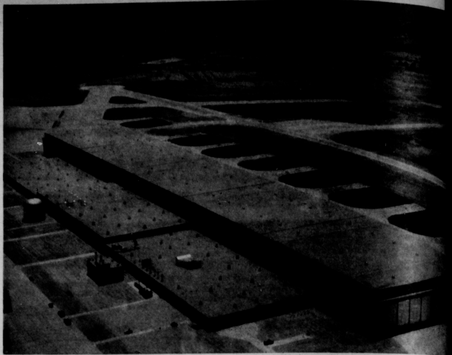
THE ROOF OF THE NEW HANGAR used for aircraft maintenance purposes resembles a runway itself as it spreads out for 2000 feet at Kelly Air Force Base, San Antonio. Twelve football games could be played simultaneously inside the 300-foot-wide hangar. The smaller shops and offices portion of the $14,000,000 project to the left is 1650 feet long and 250 feet wide.
