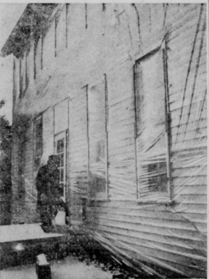
WRAPPED FOR WINTER —Wrapped in shimmering polyethylene, this old house in Lafayette, Ind., is the result of one cold winter night when the temperature fell to 10 degrees below zero. The goldfish bowl in the living room froze over, despite the fact that the oil burner was on. Purdue University Agricultural Experiment Station suggested wrapping the poorly insulated building in polyethylene film. Agricultural engineers are still testing the temperatures inside and out, but the residents of the house have been able to turn down the oil burner at night, even in coldest weather.
