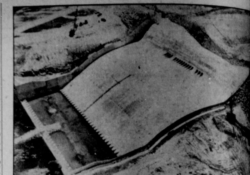
MONEY IN THE TILL —That's what water from cash register-like spillway means to neighboring farmers of Kirwin Dam, near Phillipsburg, Kan. The recently completed key unit of an 11,500-acre irrigation project, dam is 12,646 feet long, has a 400-foot-wide spillway and cost $19,500,000 to build.
