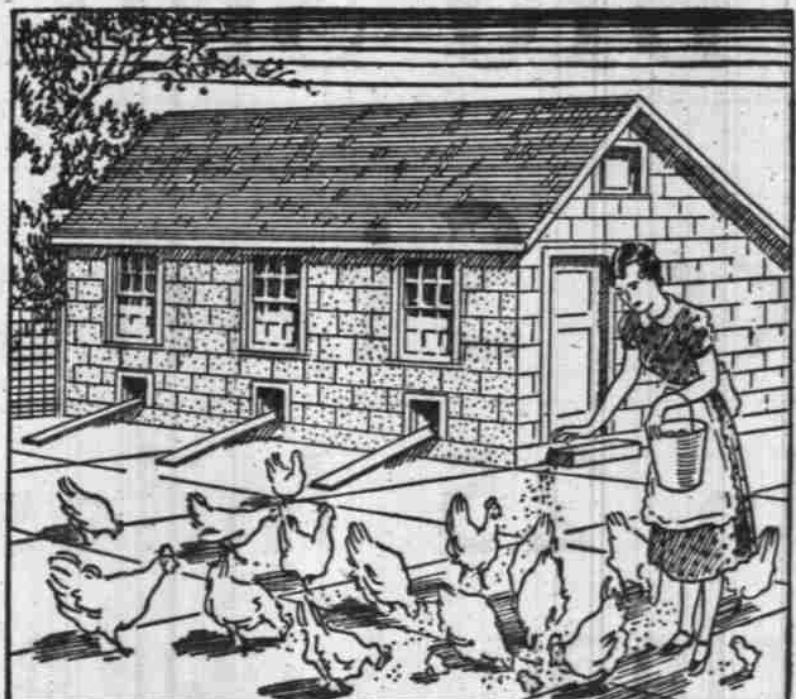
VIBRATILE HOUSES for chickens prove ideal for they are durable and fireproof and easy to keep clean. Moreover, the tile principle gives the houses insulation to protect them from any sudden weather changes and to furnish ideal conditions for high egg production. Vibratile are manufactured in Big Spring.
