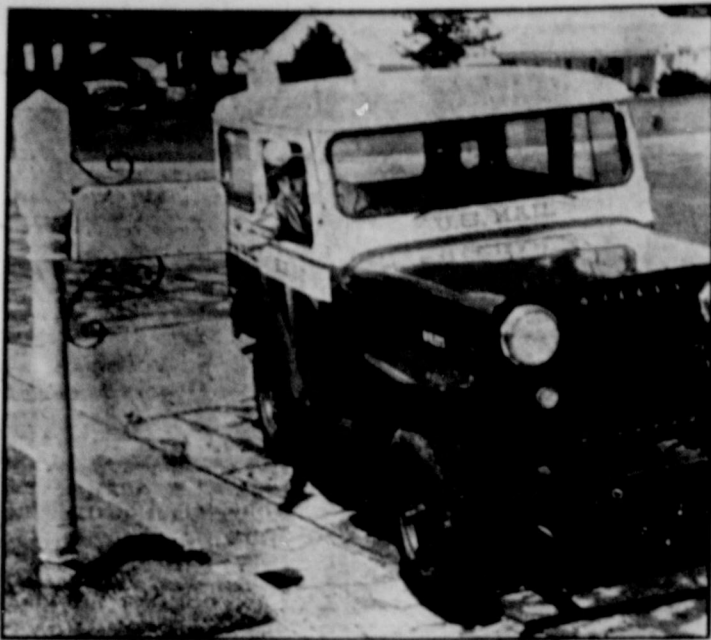
LOOK, NO WALKING —This mailman doesn't have to walk a step on his suburban route in Toledo, Ohio. That's because he's got the first American car in 30 years that features right-hand steering. The jeep, specially built for the Post Office Department, enables the carrier to drop mail into letter boxes without leaving his seat. When put into widespread use, this design promises to save the department much in time and money.
