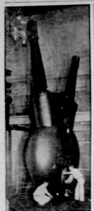
BIG CIRCUIT BUSTER-Only one of three pole units built for the world's biggest circuit breaker, the two-pronged monster seen above dwarfs three men working on it. Ready for testing, the unit was built by the General Electric Company in its Philadelphia shops.
