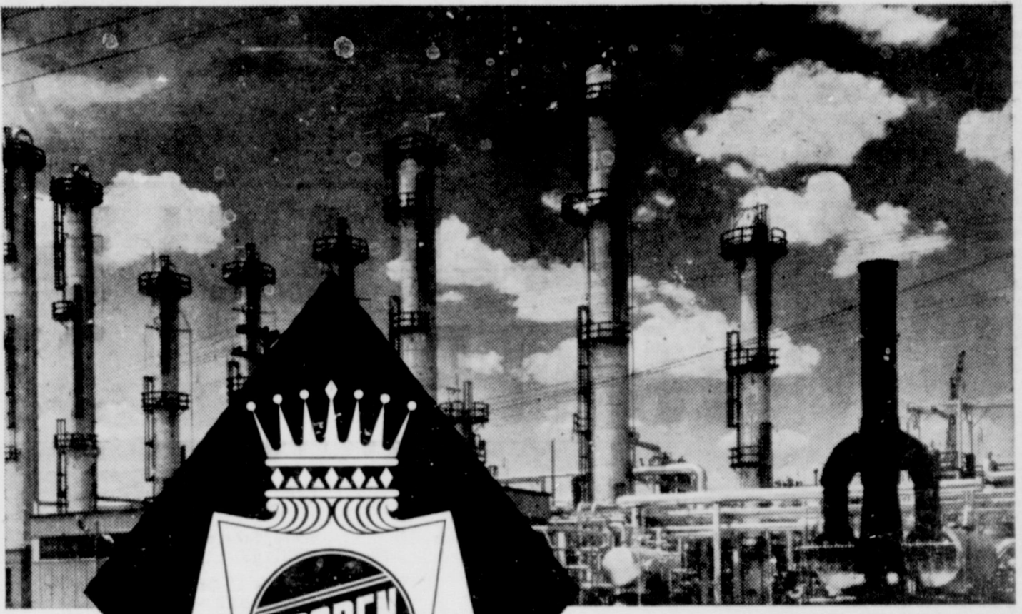
PARTIAL VIEW OF COSDEN'S MULTI-MILLION DOLLAR REFORMING UNIT
