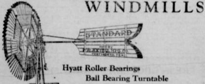
**Ball Bearing Turntable** Ring Oiling Pitman Self Tightening Wheel
