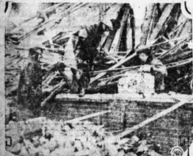
This scene of utter wreckage followed the razing of a three-story brick building—and the killing of two men—by the explosion of a huge alcohol cooking plant and still at Meadway, Pa. Seven others were injured, and searchers are pictured going through the ruins in quest of any possible victims of the tremendous blast. The man believed to have been the operator of the still escaped in a taxi-cab with the aid of two companions who held a menacing crowd at bay with drawn revolvers.
