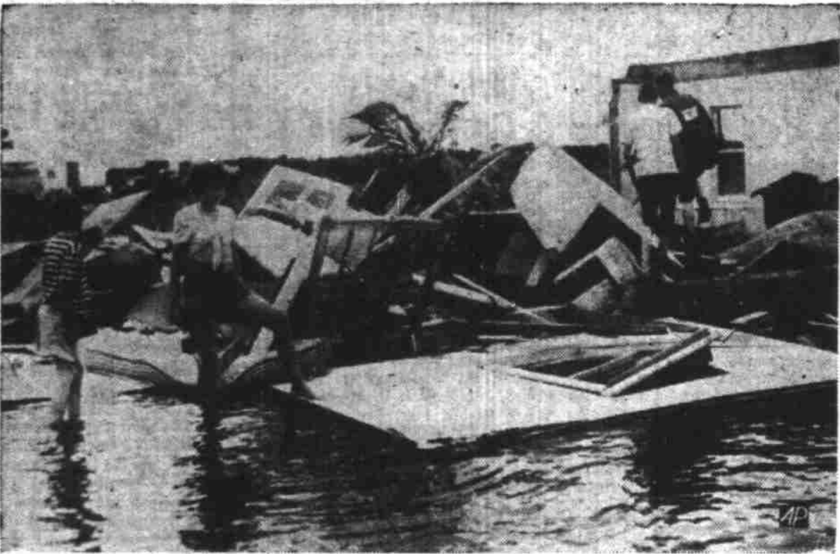
TORNADO WRECKAGE — These folks examine the remains of their home flattened by a tornado within Florida's hurricane. More than ankle deep water hampered their salvaging what was left of their belongings. (AP Wirephoto).
