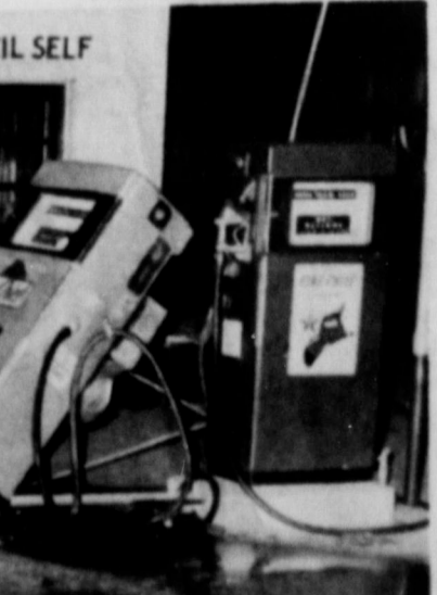
CRASH GETS STATION--A collision of two cars on 9th and Geneva Saturday night left Self's Texaco Station with heavy damage after one of the cars wound up crashing into the front of the building. Gas pumps were knocked down and a water line broke. Damage was estimated at $2,000 to the station and $5,000 for the cars. Four persons were injured in the two autos, but apparently no serious injuries sustained. (SLATONITE PHOTO)
