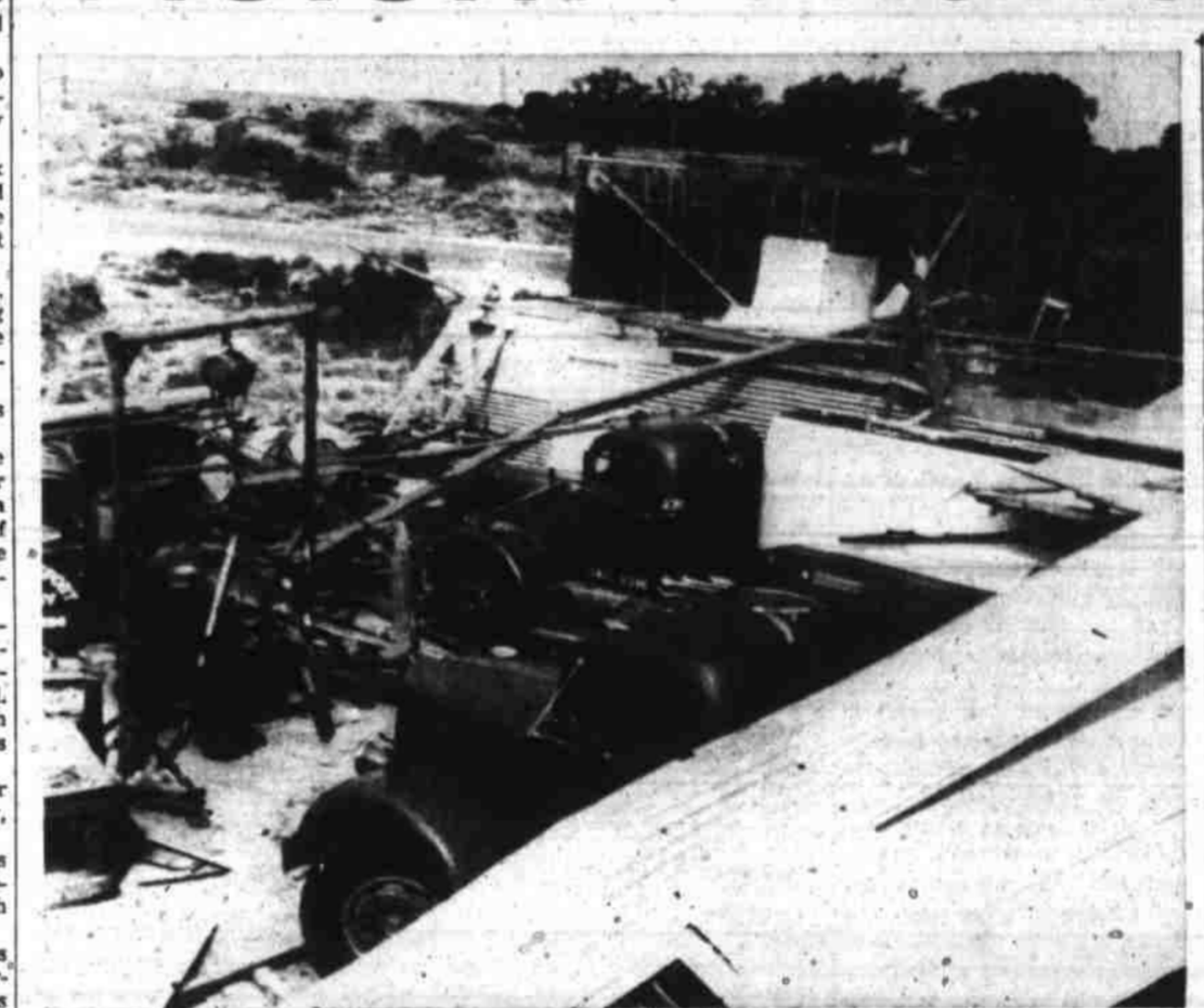
TRANSPORT FIRM'S BUILDING FALLS Winds pile roof on trucks parked in garage
