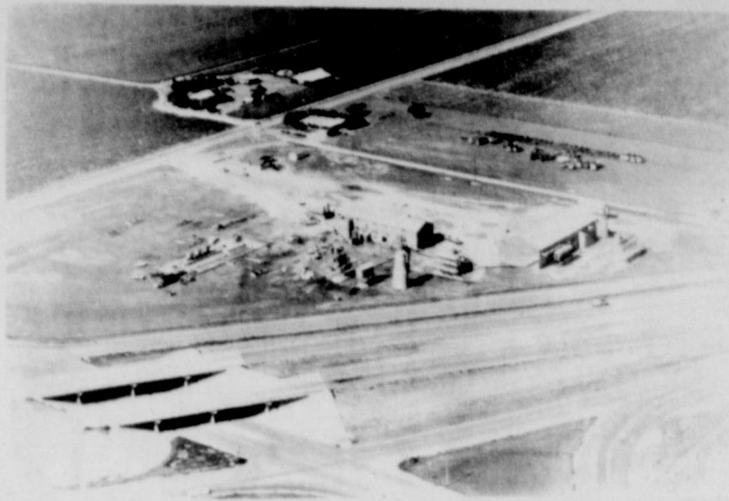
GIN MOVING PLANT---This aerial view at Slaton Co-Op Gin shows foundation being laid (middle left) for the third plant which is being moved from downtown Slaton (N. 9th St.). Present two plants can be seen in middle and at right. (SLATONITE PHOTO)
