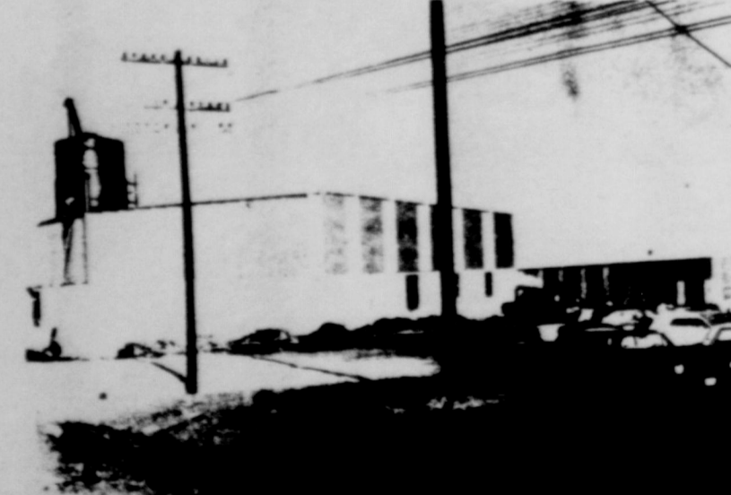
PROGRESS SEEN -- Slaton's new industry -- Modern Castings Corp. -- is beginning to take shape on the old Lubbock highway. The new plant is located across the street from Triangle Mfg. Co. Due to industrial development on the highway, a proposal has been made to officially designate the old highway as Industrial Drive. (SLATONITE PHOTO)
