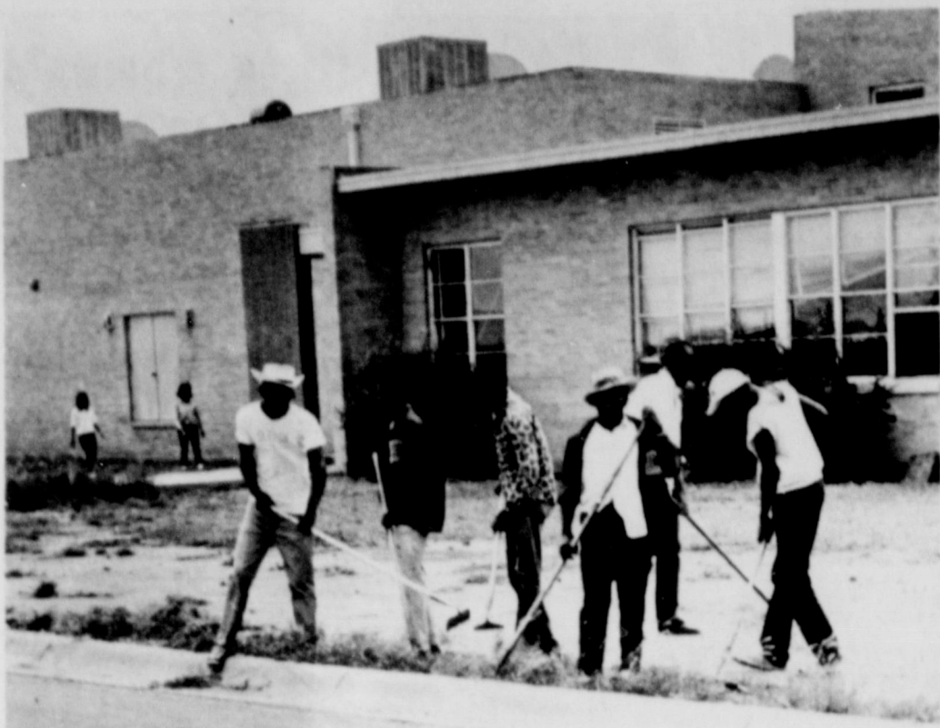
PRE-SCHOOL YARD WORK---A crew of workers were cutting weeds around Slaton High School, and other buildings, last week in preparation for the approach of the new school term. Capital improvements - including a new football stadium, gymnasium and West Ward Cafeteria - highlight Slaton school facilities. (SLATONITE PHOTO)
